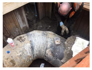
On the afternoon of the 9<sup>th</sup> April 2019, the PLCS Technical Office received a call requesting urgent assistance in the repair of a low pressure 24" steel 90 degree welded segmented bend located in a very busy area.
